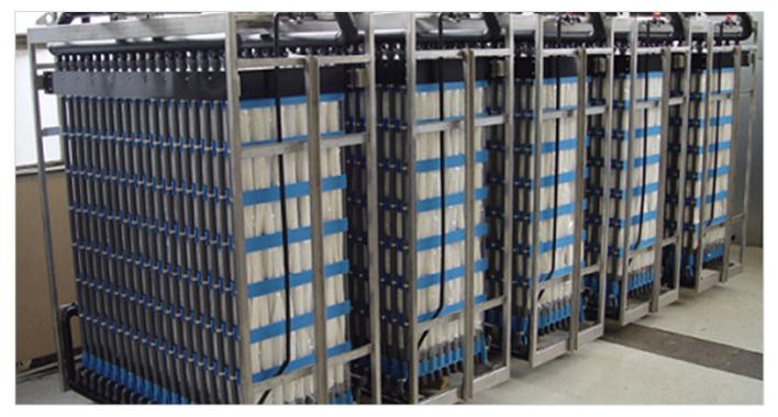
Figure 3-2 Hollow Fiber Membrane Units
