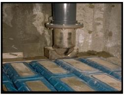
**Underdrain showing Backwash Air Header**
